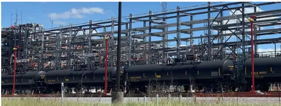
2000 GPM OSCILLATING TOWER SASOL 2016
